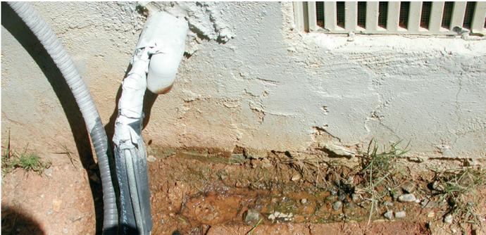
Utility access points along a building foundation are locations where pests commonly enter structures. Excessive accumulations of water should be avoided.
