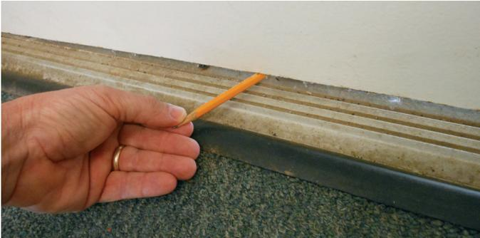
The gap under doors is a common pest entry point that can be easily sealed by installing doorsweeps.
