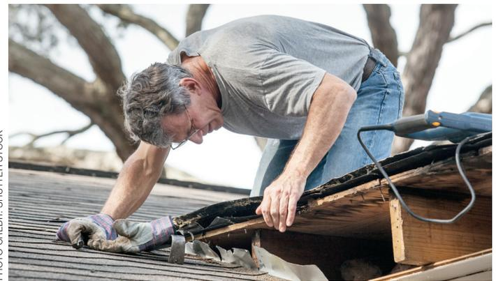
Sealing entry points on roofs is a tactic proven to reduce indoor problems with many vertebrate pests including bats, squirrels, and rats.
